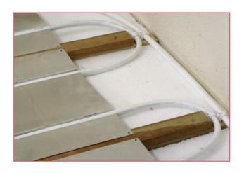
The plates are securely nailed to the top of the joists to prevent movement. The pipe work is then installed into the plates and further secured with hammer in fixings.
