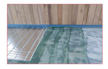
Depending on the final floor covering, an intermediate layer of self-levelling screed or timber sheeting may be required. We would offer advice on this during the initial planning stage.
